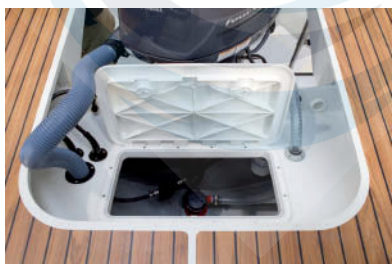
Bilge and pump access
